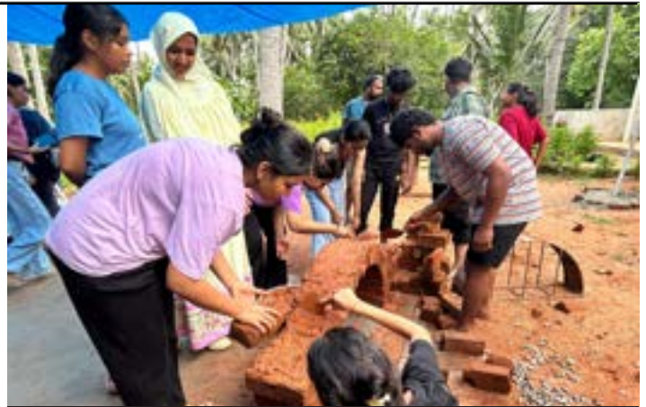
Brick Workshop, pondicherry
